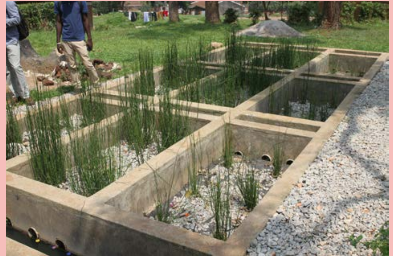
IMAGE 29 Wet Technik installation at Makerere University
